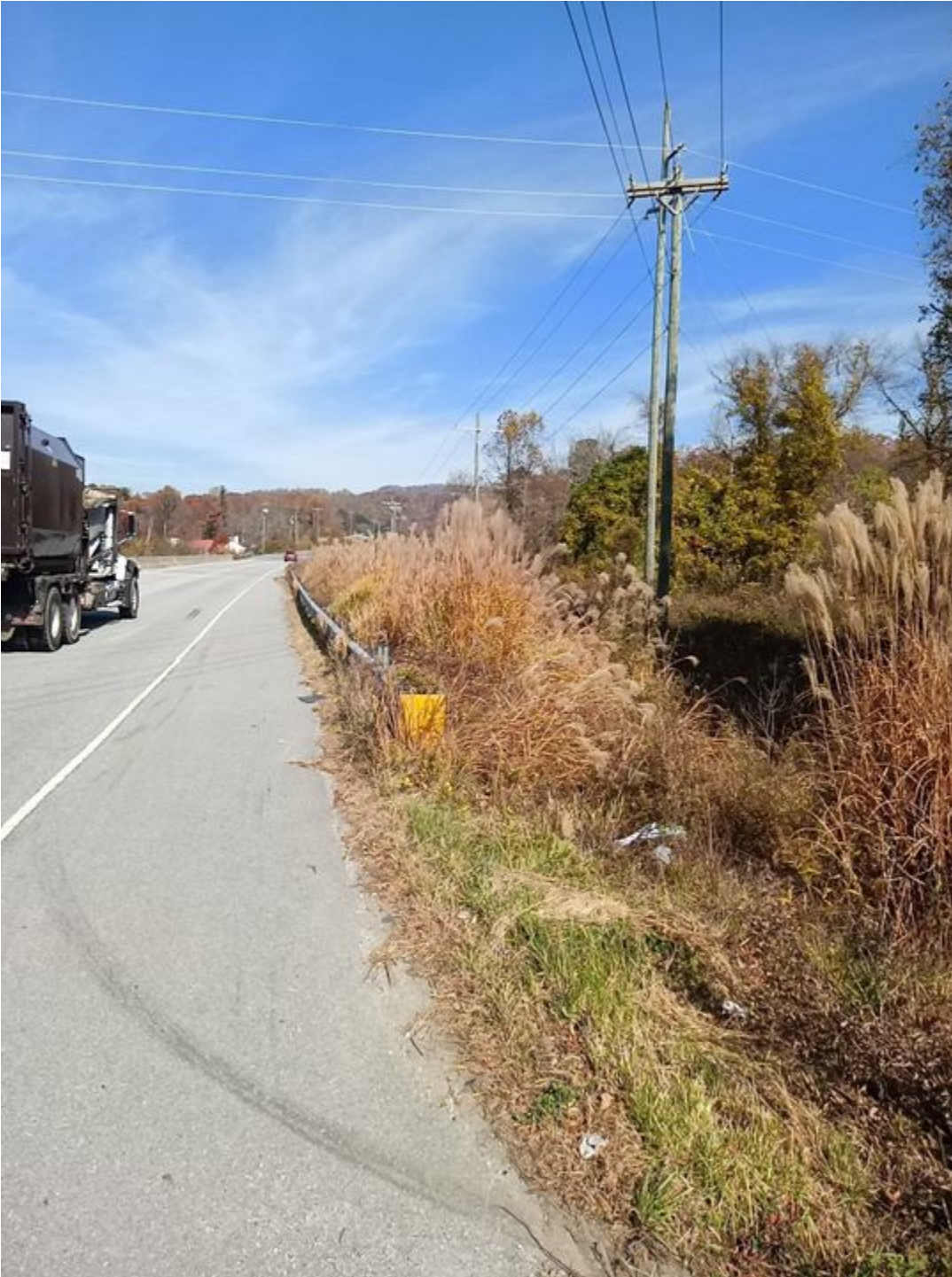
Date & Time: November 7, 2025 12:20 PM Location: 35.372105, -82.47741 Photo Direction: North
